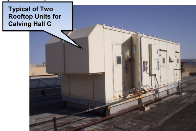
Figure 13: Calvin Hall C Rooftop Unit with Air Washer
