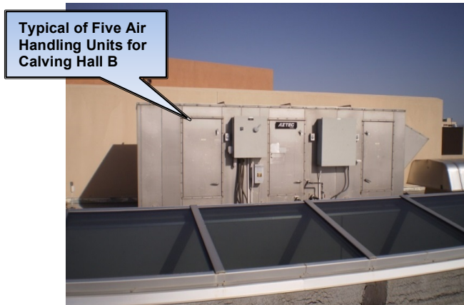
Figure 12: Calvin Hall B Air Handling Unit
